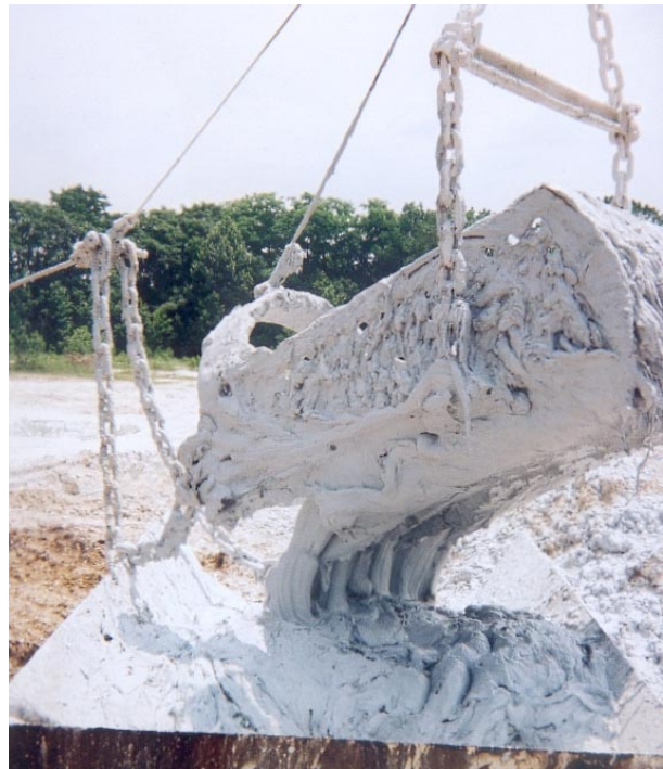
The drag line bucket dumps the sludge into the Maxcrete. The grizzly keeps large objects from entering the Maxcrete. This is primarily to protect the concrete pump.
