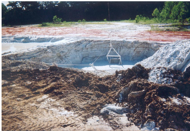
The top 3 to 5 portions of the pond have solidified, but when the material is agitated by the drag line bucket, the sludge liquefies, having the appearance and consistency of paste.
