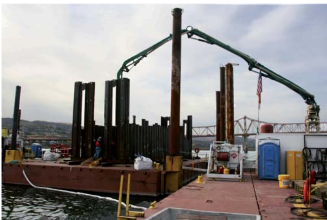
At right - Maxcrete operator feathers controls to match concrete discharge speed of Maxcrete to trailer pump. At left - 36 Meter Putzmeister Placing Boom feeds concrete over the wall of the moon pool to the divers underwater placing the rut slabs
