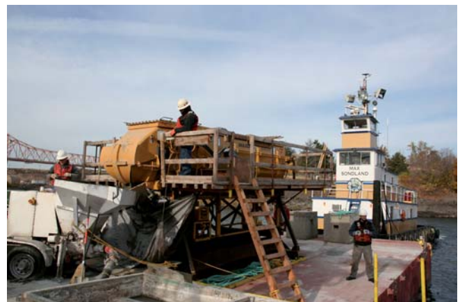
At right - Maxcrete operator feathers controls to match concrete discharge speed of Maxcrete to trailer pump. At left - 36 Meter Putzmeister Placing Boom feeds concrete over the wall of the moon pool to the divers underwater placing the rut slabs
