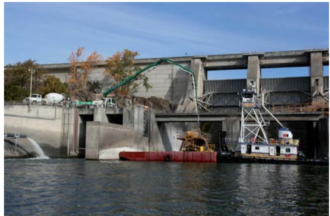
9 cubic yard truck mixers and 32 meter concrete boom truck feed concrete to barge mounted Maxcrete
