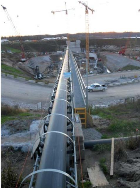
The overland belt conveyor system consisted of 600' (182m) of standard conveyor with supports every 32' (10m), and 600' (182m) of truss conveyor with supports every 98' (30m).
