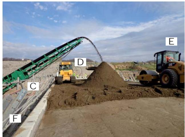
Maxon Surgecrete (A) accepts soil cement from end dumps (B) while continuously feeding telestacker (C) during construction of left and right embankments. A dozer (D) and soil compactor (E) distribute and compress each lift. The face of the embankments were protected with precast panels (F) for upstream erosion control.
