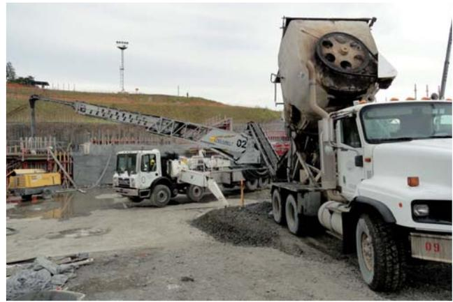
Walsh utilized truck-mounted Maxon Agitors and a truck-mounted Putzmeister TB 130 to transport and place concrete on lower level foundation and mat pours.
