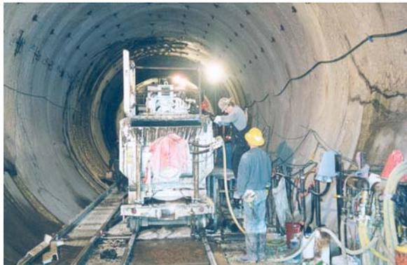
*Maxcrete awaits next set of Agitators while feeding consistent supply of concrete to the pump*
