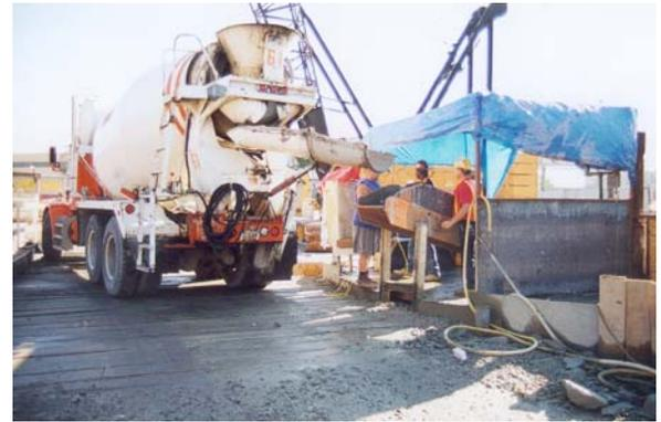
*Concrete delivered to site, fed to drop pipe*
