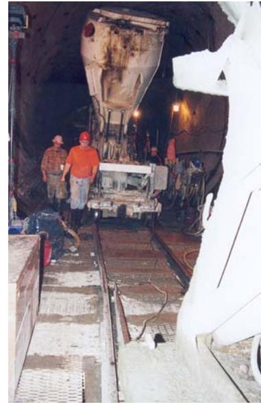
*1<sup>st</sup> Agitor discharges into Maxcrete, while tow cable is run to 2<sup>nd</sup> Agitor (at far right)*
