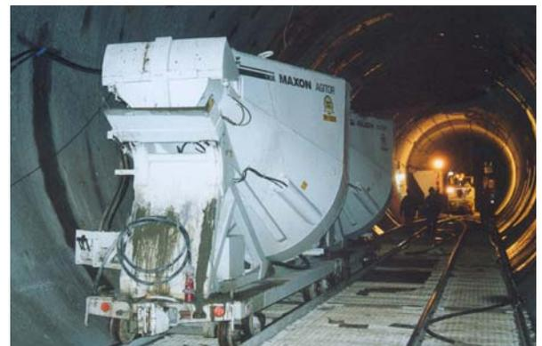
*1<sup>st</sup> and 2<sup>nd</sup> Agitor after discharging full load, wait on bridge for 3<sup>rd</sup> Agitor to complete*
