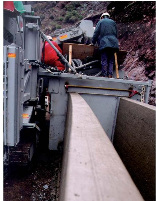
*The concrete channel is slipformed from the Power Curbers 8700.*
