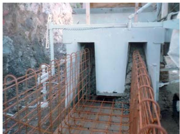
*Front view showing the steel rebar as the slipform pours concrete into the channel forms*
