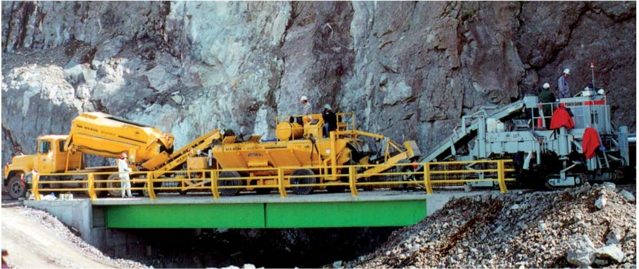
*Truck-Mounted Maxon Maxcrete transporter (left) feeds Maxon Mobile Maxcrete (center) which then feeds the Power Curbers Slipform (right). Narrow pathways and height restrictions mandated the use of low profile Maxon equipment.*
