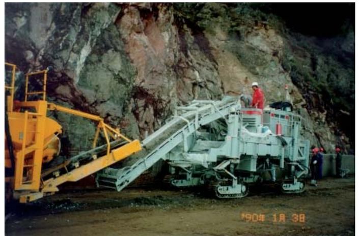
*...to the Power Curber 8700 Slipform Paver forming the channel*
