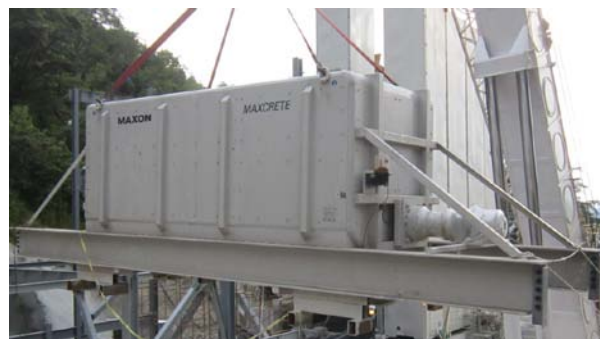
Maxon 20 cubic meter capacity paste mixer during installation at Escobal Silver Mine in Guatemala.
