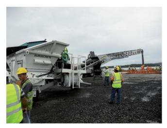
From the Surgrecrete's platform, the operator can view the Maxon Agitors discharging into the Surgecrete hopper and the concrete feeding to Putzmeister Telebelt, thus ensuring quality concrete throughout the delivery process.
