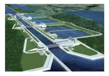
Computer rendering of completed Panama Canal lock addition. The new locks will run parallel to the existing Canal/ Locks and offer a third lane and set of locks for today's larger vessels.
