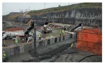
12 cubic yard Maxon Agitors transport and feed large aggregate (3"+) concrete to two (2) Putzmeister TB130 Telebelts for construction of the lock chamber floor.
