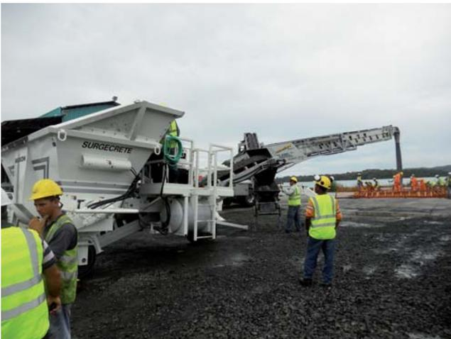
From the Surgecrete's platform, the operator can view the Maxon Agitors discharging into the Surgecrete hopper and the concrete feeding to Putzmeister Telebelt, thus ensuring quality concrete throughout the delivery process.
