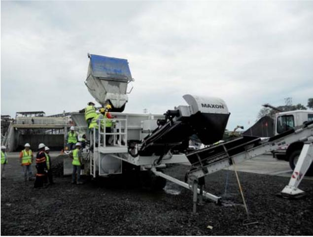
Maxon Agitor equipped with the Hi-Dump chute discharges complete load directly into the Maxon Surgecrete, which meters concrete to the Putzmeister Telebelt.
