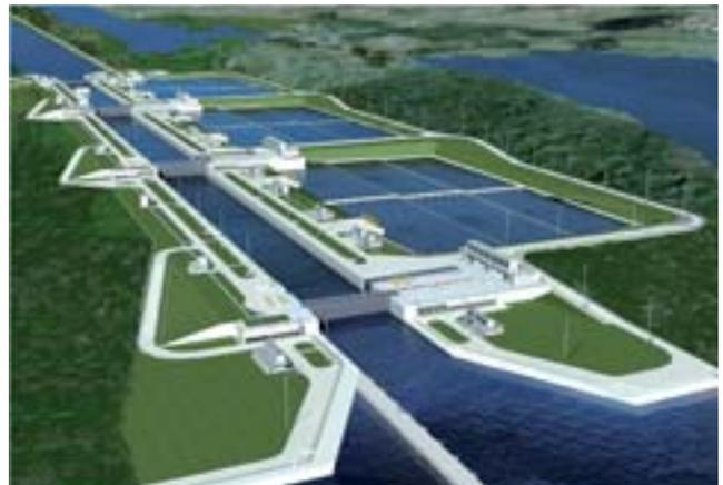
Computer rendering of completed Panama Canal lock addition. The new locks will run parallel to the existing Canal/Locks and offer a third lane and set of locks for today's larger vessels.
