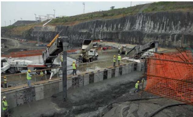
12 cubic yard Maxon Agitators transport and feed large aggregate (3"+) concrete to two (2) Putzmeister TB130 Telebelts for construction of the lock chamber floor.
