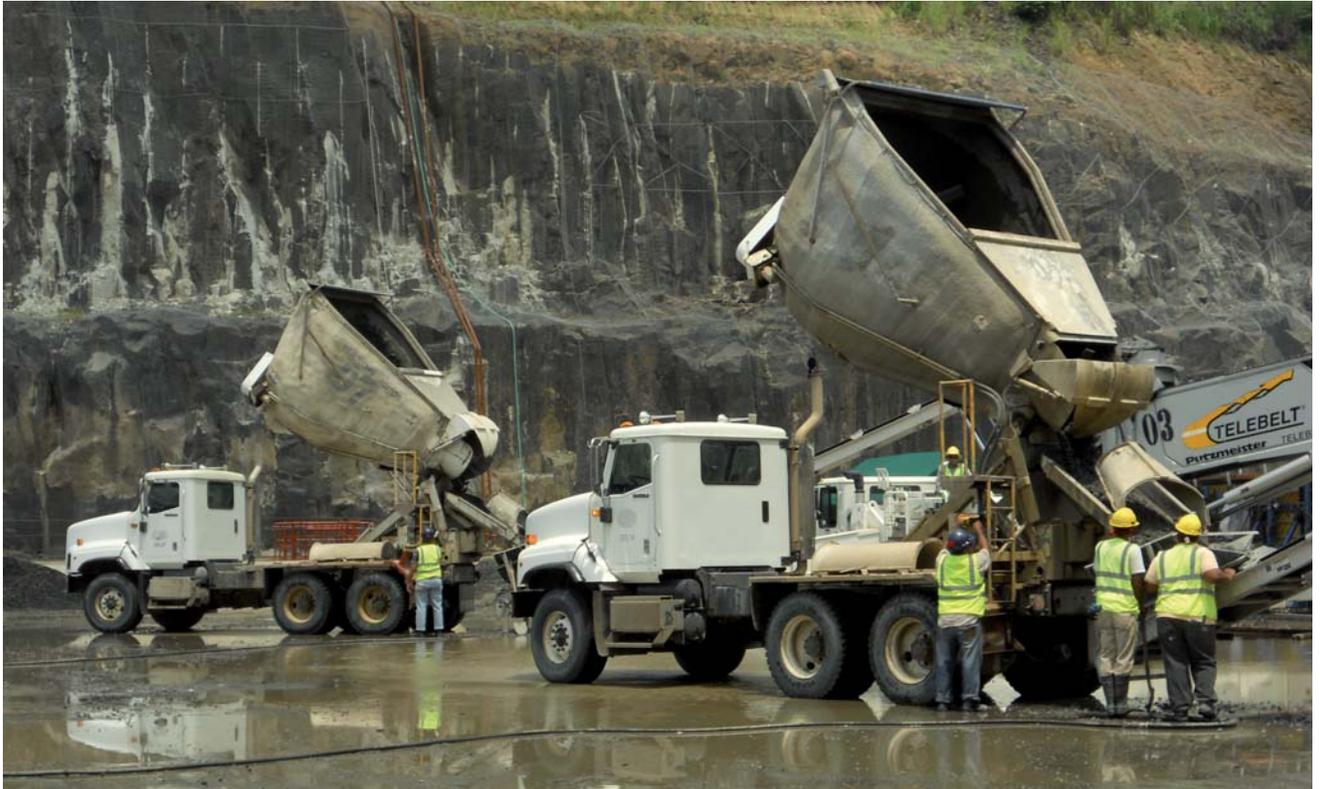
Two (2) 12 cubic yard Maxon Agitators feed large aggregate concrete to two (2) Putzmeister TB130 Telebelts. Combination rollback/steel covers on the Agitators allow operation in areas of Panama where annual rainfall can exceed 120"/year.
