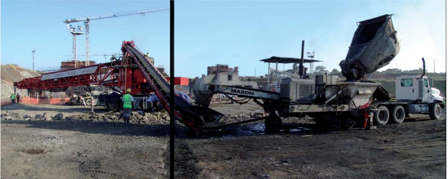
*Above: Mobile Maxon Surcrete accepts concrete from truck mounted Maxon Agitors while simultaneously feeding Putzmeister Telebelt.*
