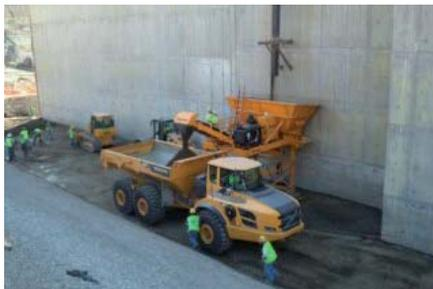
*Left: Stationary Surcrete at hydroelectric project continuously accepts soil cement from pugmill above while feeding dump trucks.*
