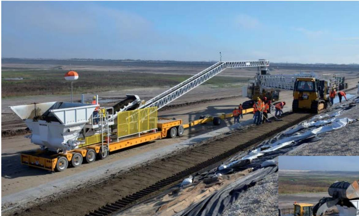
*Above and right: Trailer-Mounted Surcrete accepts soil cement while simultaneously feeding 24" charge belt of Crawler Placer allowing continuous placing.*
