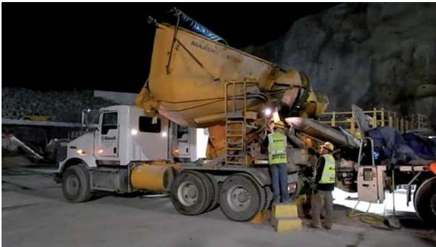
Dump operator controls hoist/concrete discharge of Maxon Agitor to boom pump hopper (while the next Agitor moves into position to ensure continuous concrete supply to the pump hopper)
