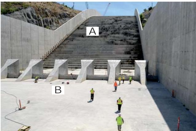
Engineers inspect the completed Spillway Chute and the six concrete monoliths in the Stilling Basin designed to slow water flow before discharging into the American River.
