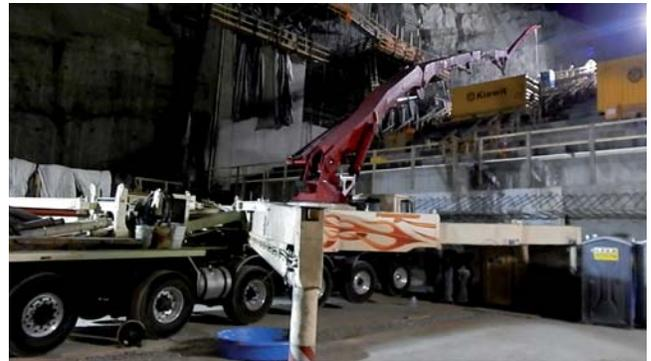
Kiewit utilized 50 and 60 meter class Putzmeister concrete boom pumps to reach the upper regions of the Spillway Chute from the base of the Stilling Basin.
