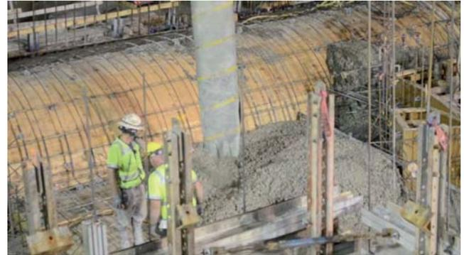
Above: For the Control Gate construction, Granite's Agitators discharged directly to truck-mounted belt placing conveyors. 5' concrete lifts were poured during the night to maintain the temperature of the chilled concrete.
