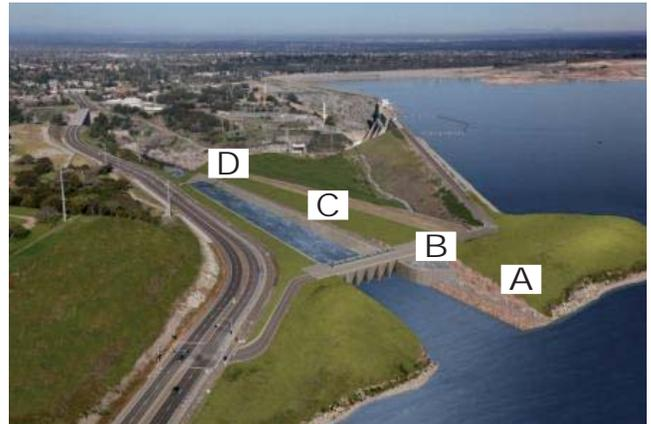
Completed Project Rendering: 1,100' Approach Channel (A), 6-Gate Control Structure (B) 3,000' Spillway Chute (C), and Stilling Basin (D).
