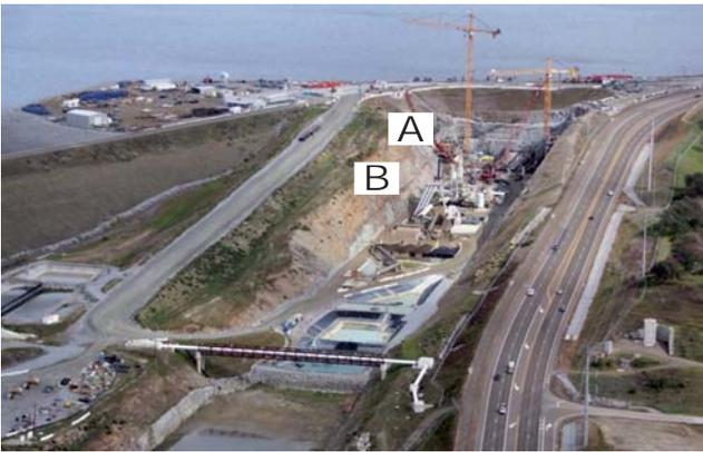
Excavation complete, Granite begins construction of the Control Gate (A). The concrete batch plant (B) was set-up temporarily in the spillway to reduce transit distances.
