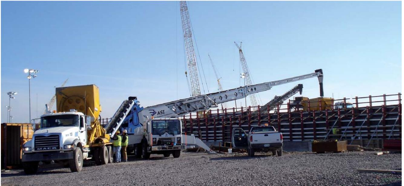
*Agitators were used in conjunction with Telebelts for direct placement of Roller Compacted Concrete (RCC) and Conventional Vibratory Concrete (CVC).*
