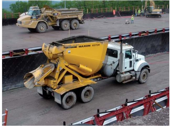
Truck-mounted Agitator driving on RCC dam surface, returning for load.
