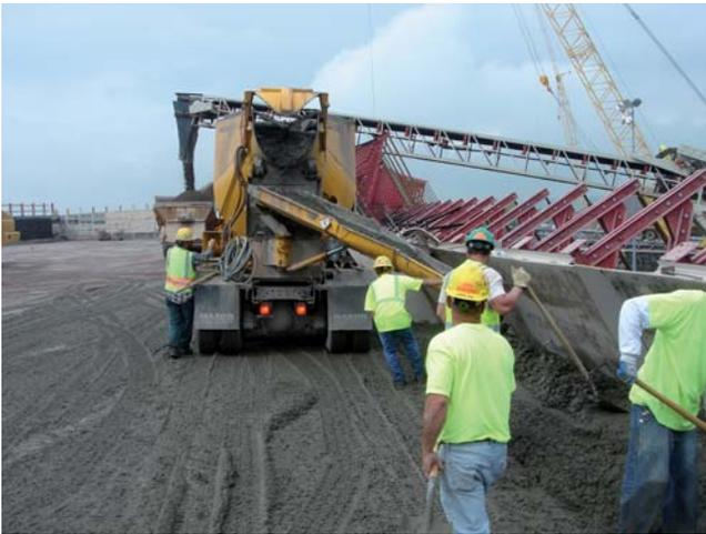
Agitator discharging grout enriched RCC directly adjacent to the dam face formworks.
