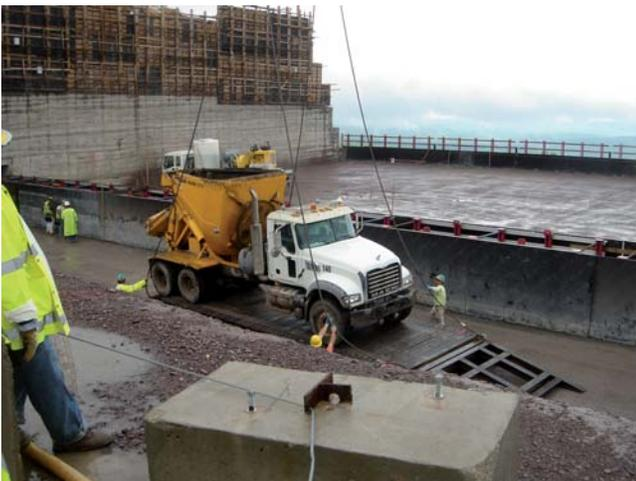
Agitator was lifted from one RCC section to the next with a special platform and crane.
