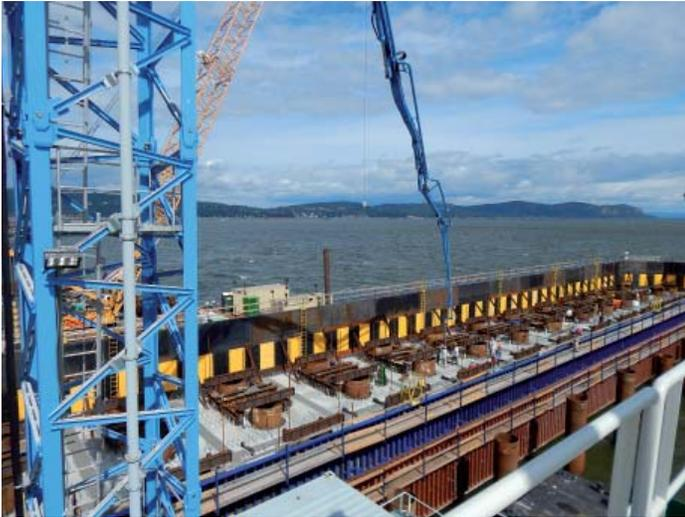
In early July 2014, the first concrete production/placing barge was put into service, supplying the concrete for the structural support piling caps. The bridge will require over 1,000 steel tubes/pilings each filled with steel reinforced concrete and then tied together with concrete caps. During initial bridge construction, TZC is building the bases that will support the main 419' towers.
