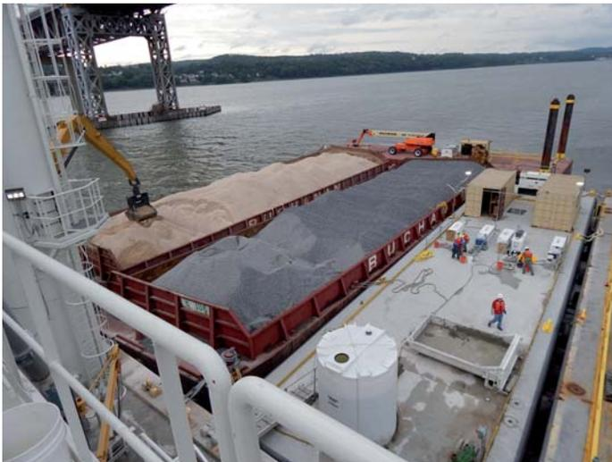
Just up-river from the project site, material supply barges are loaded from shore with sand, aggregate, cement, flyash, slag and water. To maintain the high volume concrete production, each concrete plant/placing barge is equipped with a Cat excavator to rapidly offload the sand and aggregate from the material supply barges to the concrete plant bins.
