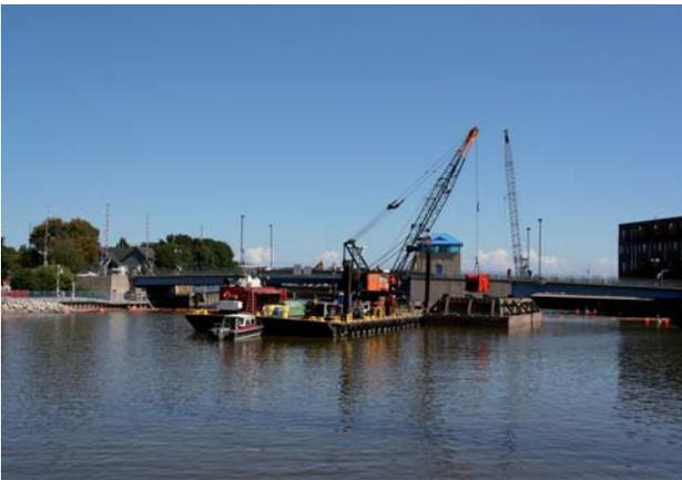
*Barge-mounted crane excavator with dredge bucket excavates contaminated sediment from the Sheboygan River. Soils are barged up river to the processing site.*
