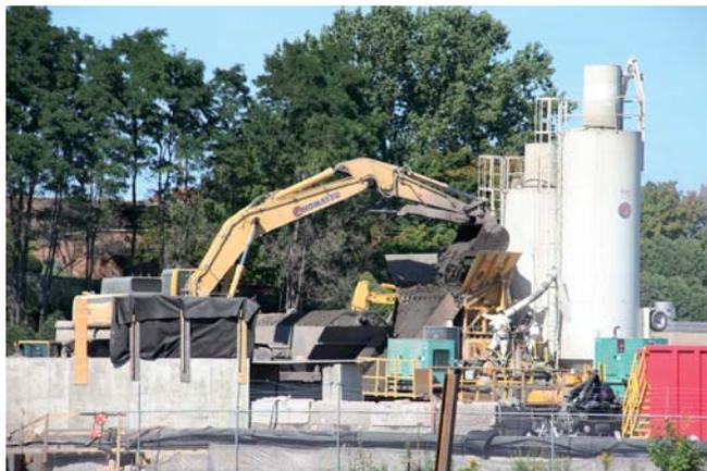
*Hydraulic excavator feeds sediment to grizzly screen mounted above the 16 yd Maxcrete. The grizzly prevents large foreign material dredged from the river bed (tree stumps, etc) from entering and stalling the agitator in the Maxcretes.*
