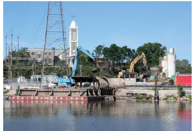
*Material handler (at left) transfers sediment from barge to concrete pad on the processing site. Hydraulic excavator (at right) then feeds soils to the grizzly and mixers.*
