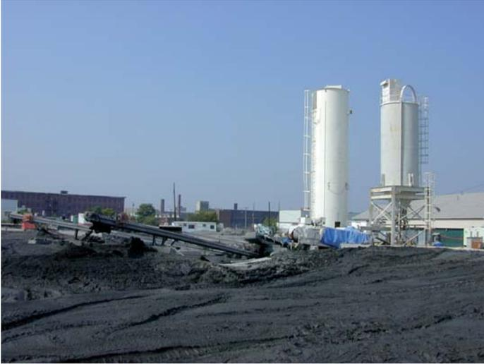
At a former brownfield site directly adjacent to the harbor, Dry Dredge erected two silos, the Maxcreters and conveyors to mix the dredged soils with the reagents. Prior to starting the job, Dry Dredge poured three concrete pads onto which the mixed materials could be dispersed and allowed to dry.
