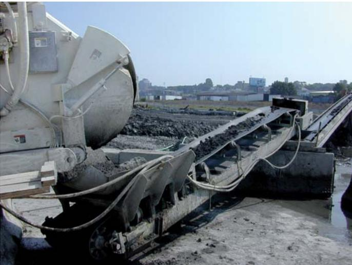
Above: The Maxcrete was fitted with a 20' discharge conveyor that could be swung to hit one of the three 50' placing conveyors.
