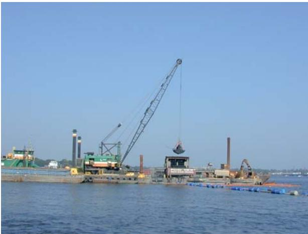
Barge-mounted crane excavator with dredge bucket excavates contaminated soils from the harbor. Soils are screened and pumped 1400' to shore via floating pipe line.
