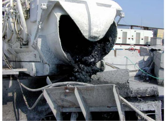
The large hydraulically operated discharge gate of the Maxcrete allowed the contractor to open/close the gate to adjust the retention time in the mixer depending on the moisture content of the excavated soils and the volume of solidifying agent.
