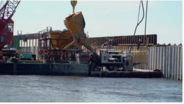
Each of the three barges included two 10 yard Agitors with elevated platform to allow a single person to operate both units from a single position. The platforms also allowed the Agitors to discharge directly into the barge mounted concrete trailer pumps (see photo left). While two Agitors were being loaded at shore, a second barge would be in transit to/from the placing site, while the third set of Agitors was feeding the trailer pump on the barge.
