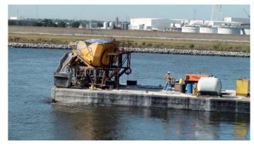
Above: Maxon Agitors were fed from redi-mix trucks on shore. Each open-top Agitor was equipped with combination steel/roll back covers for fast loading and consistent quality concrete even in wet/hot conditions. The Agitors were powered with an indepedent diesel power pack allowing the Agitors to agitate the concrete while in transit for the 1+ mile trip to the placing site, ensuring quality concrete with every load.
