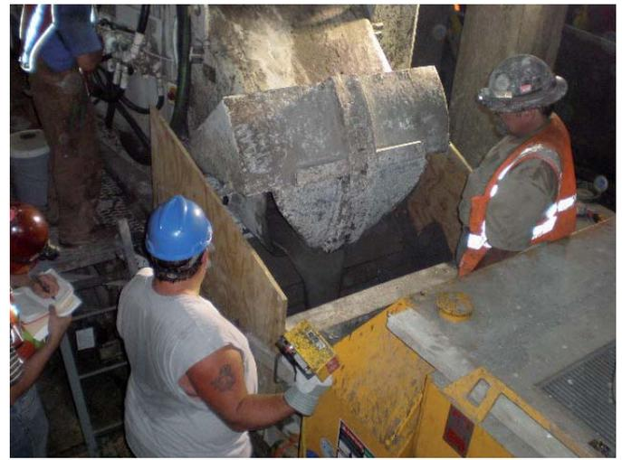
The electrically powered Maxon Maxcrete was supplied with an operator's platform with controls for both the Maxcrete and the pump. From this position a single operator could view both the inside of the Maxcrete and the pump hopper while operating the controls, which reduced the number of operators required on the job.
