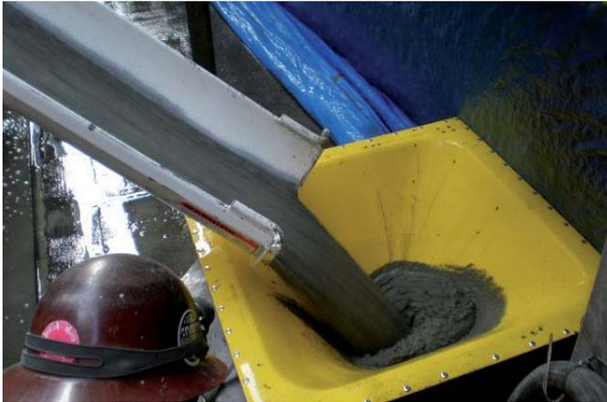
Redi-mix concrete was delivered to the corner of 52nd Street and Park Avenue, the most expensive real-estate in the world, by Ferrara Bros. Building Materials Corp. in 10 yard transit mixers. The concrete was then chuted below ground approximately 140 feet to the Maxcrete positioned on the subway rail siding. With the Maxon Maxcrete surge hopper continuously mixing and feeding the concrete pump below ground, the redi-mix trucks could discharge their entire load without delay.
