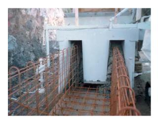
Front view showing the steel rebar as the slipform pours concrete into the channel forms
