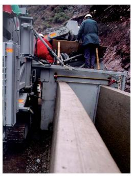
The concrete channel is slipformed from the Power Curbers 8700.
