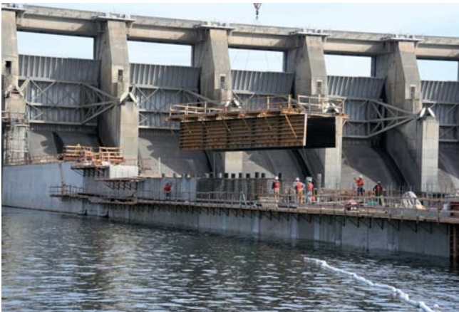
Precast caps are lowered into place during the final stages of the wall construction.
