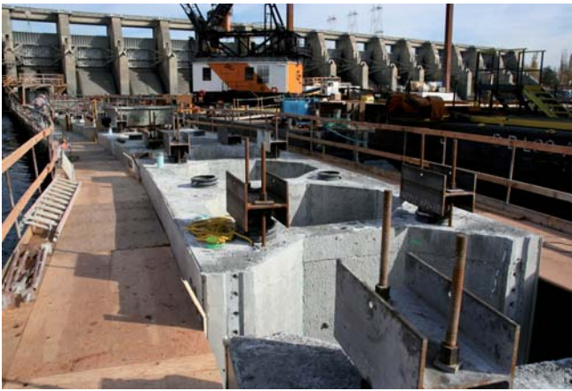
Top of precast section visible above the water line are tied into rut slabs below
